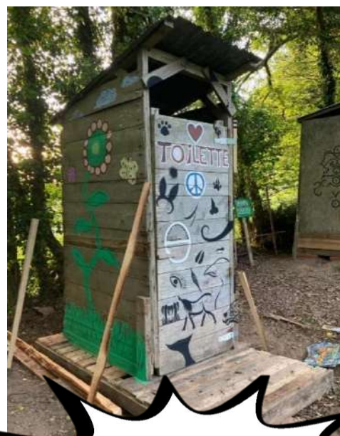
Figure 32. Toilettes sèches, Guingan.
